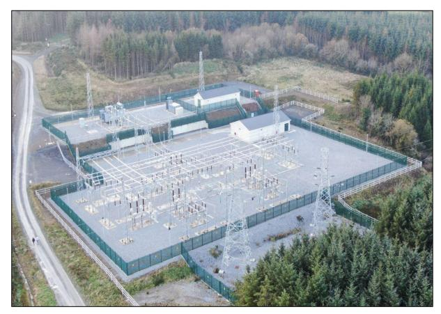
Figure 3.3: Example of a 110kV AIS Substation with split-level design
